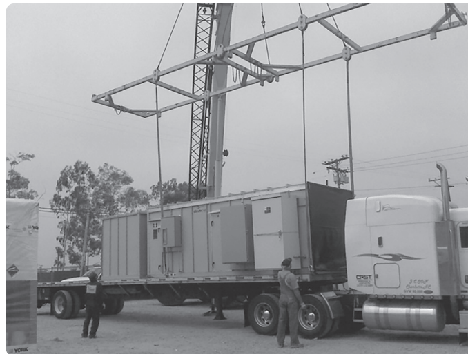
Figure 8: Example of Proper Rigging and Lifting 2
